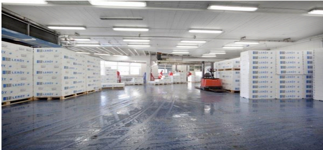
AcryliCon Décor System installed in 2004, Austevoll Fiskeindustri AS in Norway, Picture taken in 2010.
